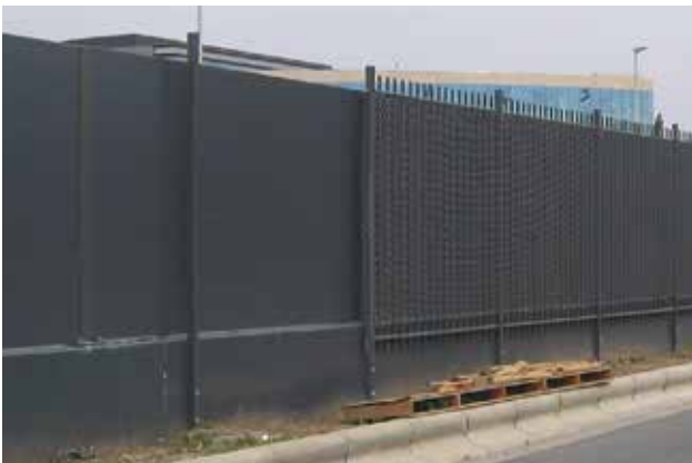
Absorbent noise panels with screens along highway E18, Oslo, Norway.
