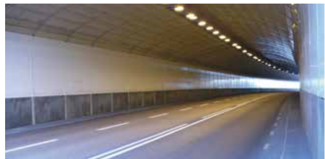
Powder-lacquered noise panels, Lindö Tunnel, Stockholm, Sweden.
