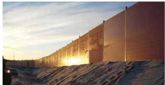
Noise panels along highway E10 at discharge station for iron ore, Svappavaara, Sweden.
