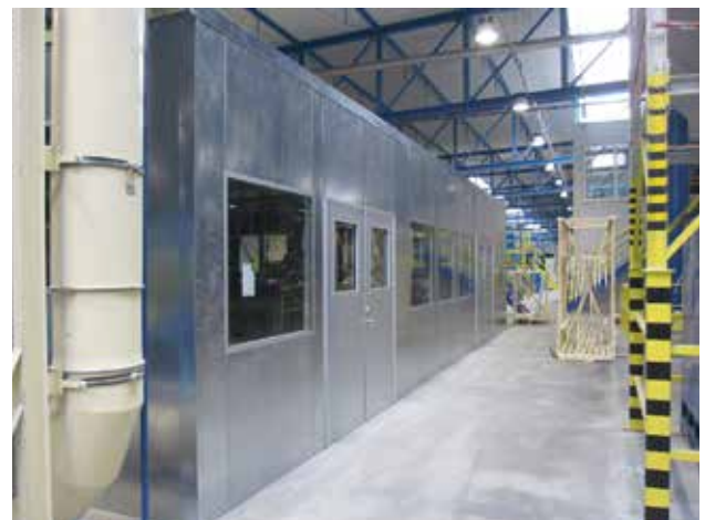
Noise enclosure, Teplice, Czech Republic.
